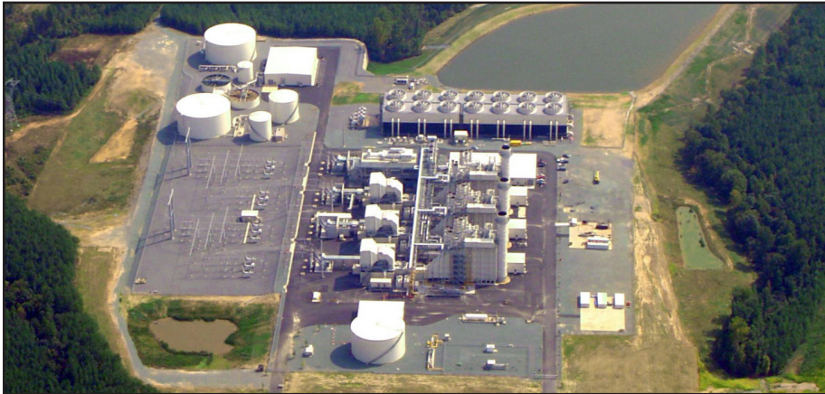
The 885 MW Tenaska Virginia Generating Station near Scottsville, Va., is a natural-gas fueled plant that produces electricity in an environmentally responsible manner.
